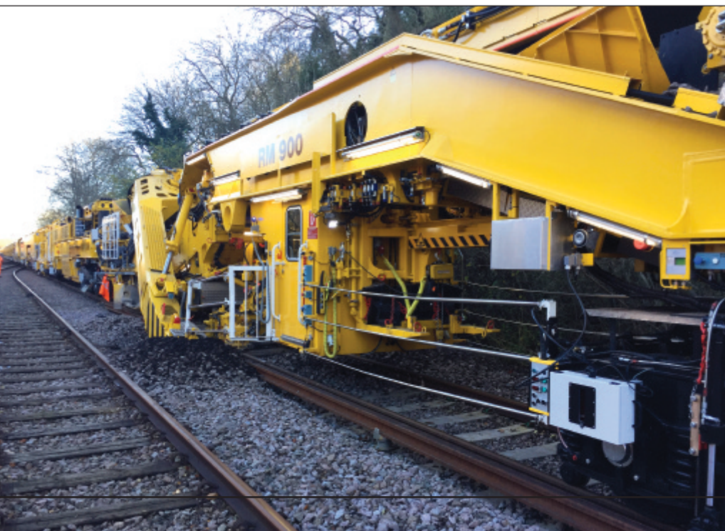
Left: The USP 5000 ballast regulator in action at the RIDC.
